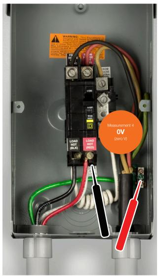
If measurements 1 - 4 are inaccurate, the service voltage is faulty. Call an electrician.
